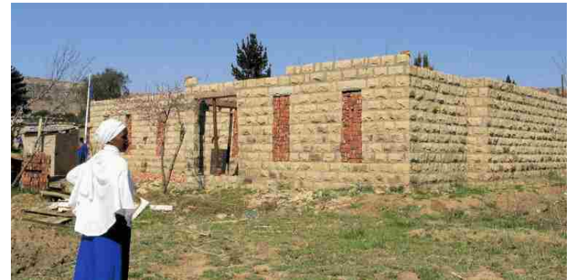
The walls on the new building
